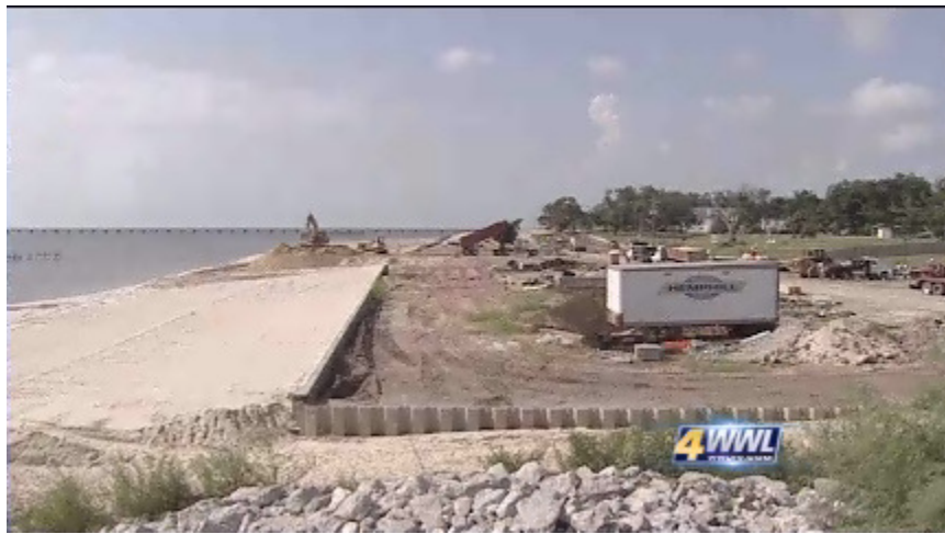
The new Bay St. Louis seawall stands 12 feet tall from the base of the sand, 20 feet above sea level at the top of the wall. Bay St. Louis Mayor Les Fillingame praised the corps for their efforts, because he said the new seawall accomplishes three missions. He called it "beautiful," "functional," and he said it would provide the necessary storm surge protection. WWL TV report dated August 12, 2011
